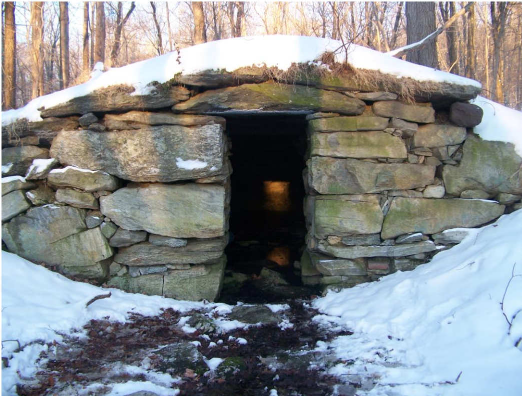
Figure 2: Corbelled Stone Chamber Found on the Brown-Barrett Farm, with sunrise on the solstice shining through the opening.
