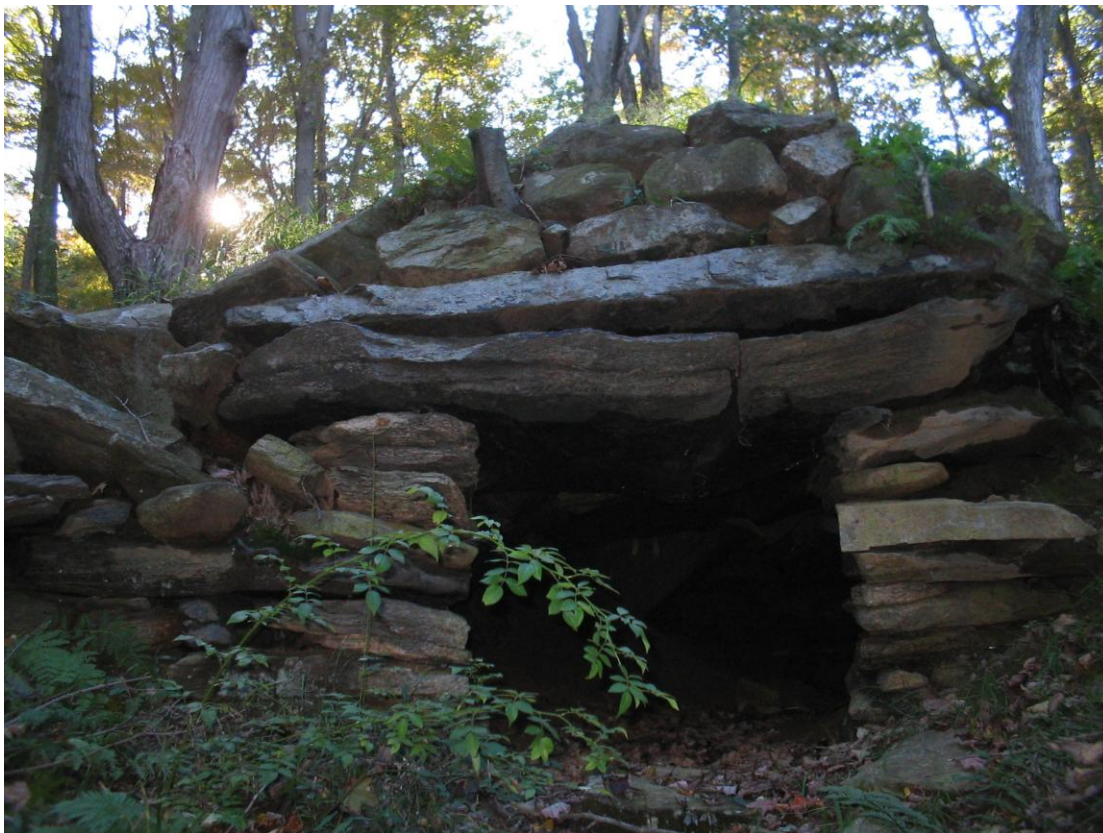
Figure 3: Corbelled Stone Chamber with Cracked Lintel Stone
